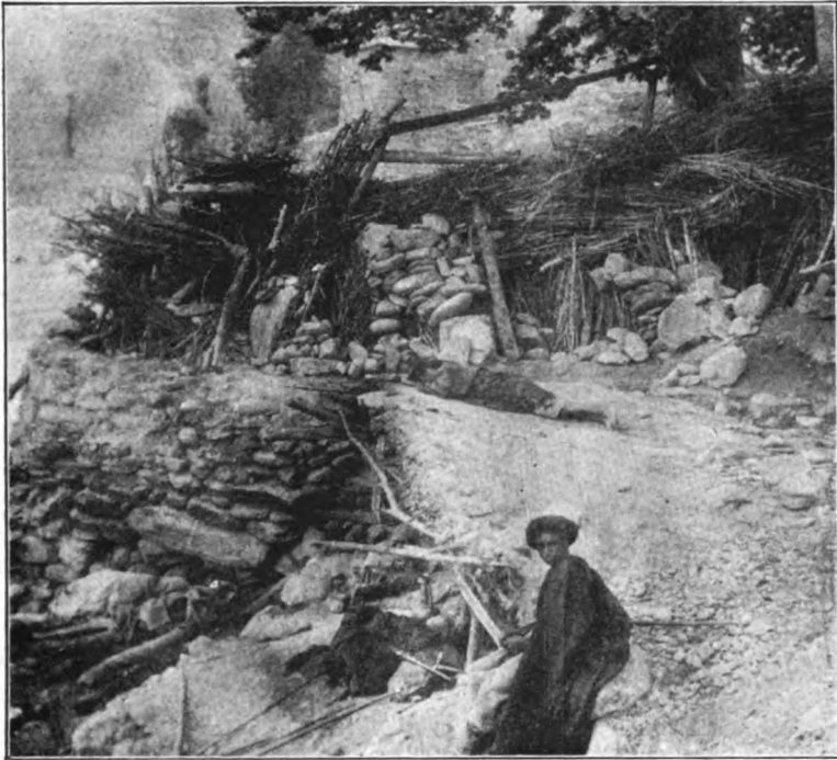
DEMOLISHED SUMMER-HOUSE WITH LOWER PART OF THE GUN TOWER IN THE BACKGROUND.
